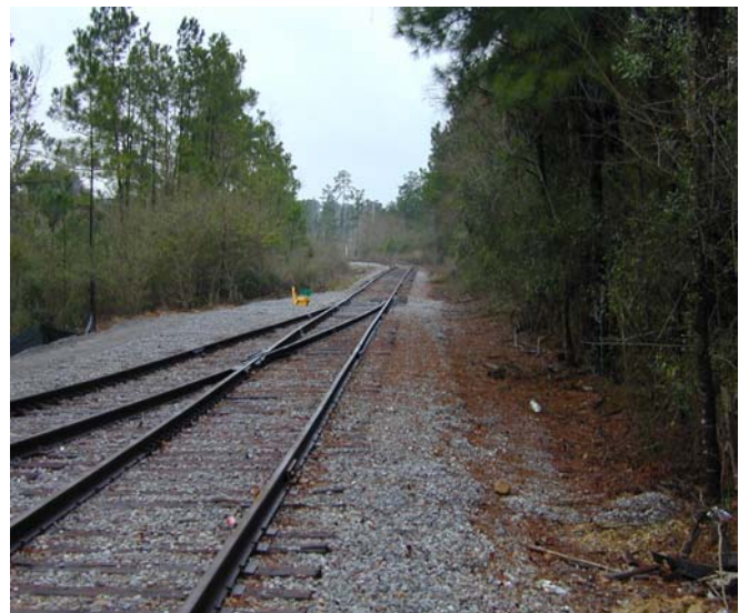
Railroad spur in Tangipahoa Parish partially funded with EDAP funds.
