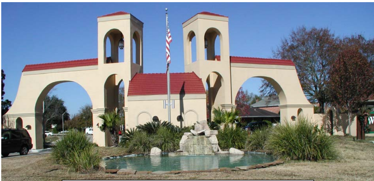
Renovated Entrance Structure - Woodlake Estates Subdivision
