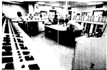
Central Control distributes electrical power to water, sewerage and drainage facilities throughout the city.
