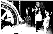
Martin Lancaster, assistant secretary of the Army for civil works, tours Deshaige Pumping Station One as part of a U.S. Corps of Engineers federally-funded public works program.
