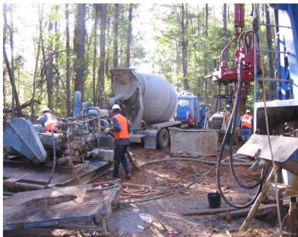
Exhibit 18 Site Restoration Project
