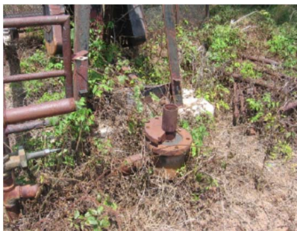
Exhibit 9 Abandoned Inactive Well Still in Active Status in SONRIS
